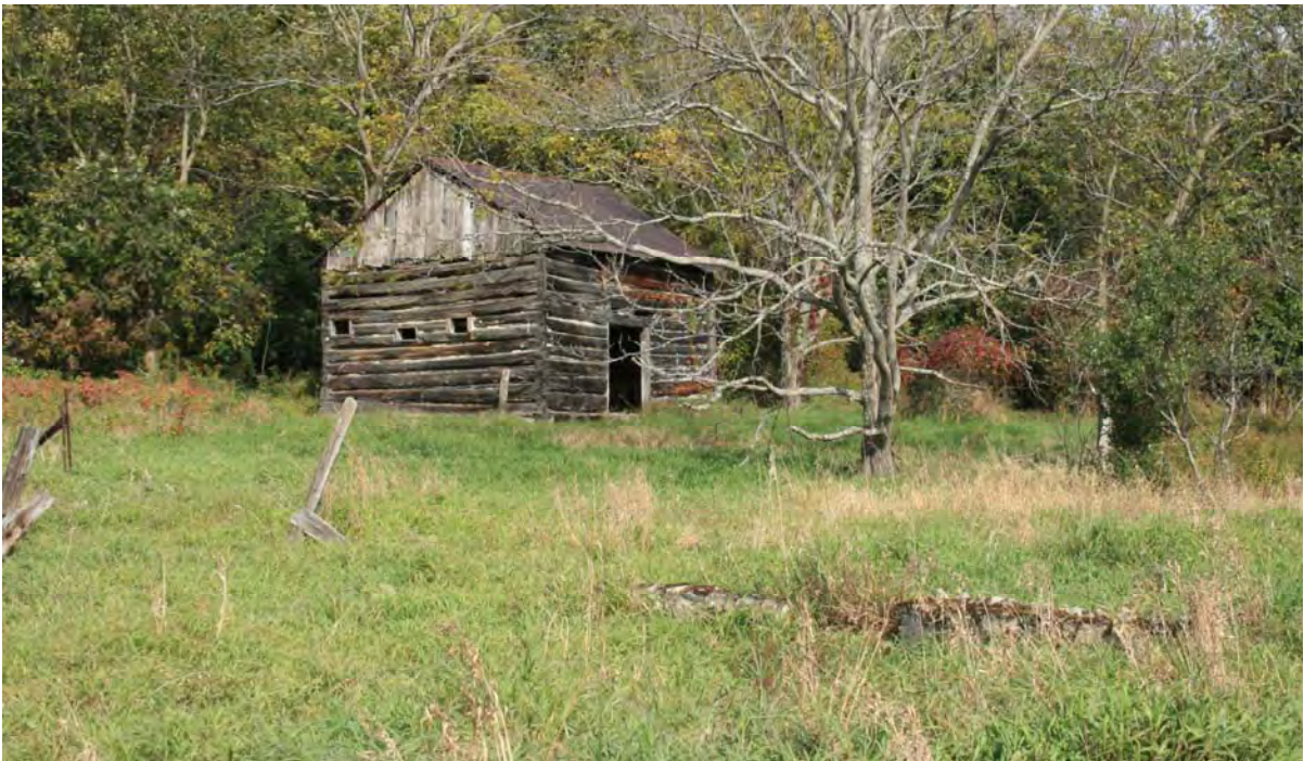
PLATE 7: Standing log barn (Log Structure 2) with concrete foundation in foreground located just outside of Site B in Lot 9, Concession I. Looking southeast. September 26, 2009.
