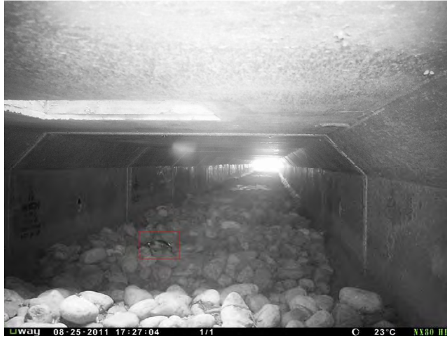
Plate 2. A Blanding's turtle moving through culvert CV6 that carries East Shirleys Brook..
