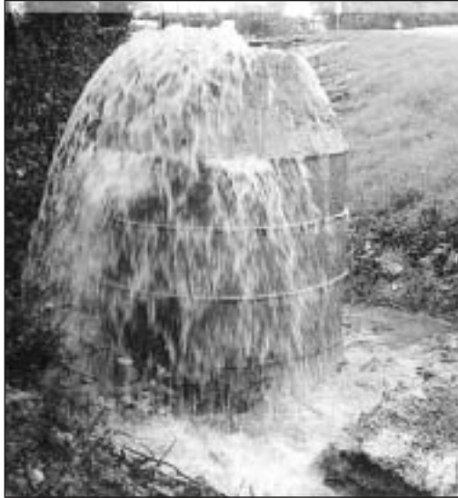
Overflowing sewer manhole
