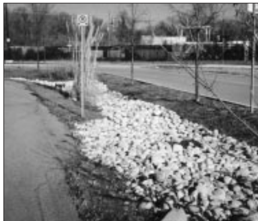
Engineering standards have to be changed to allow for alternatives to roadside ditches
