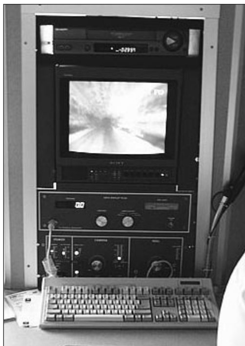
Closed circuit television (CCTV) used to inspect sewers
