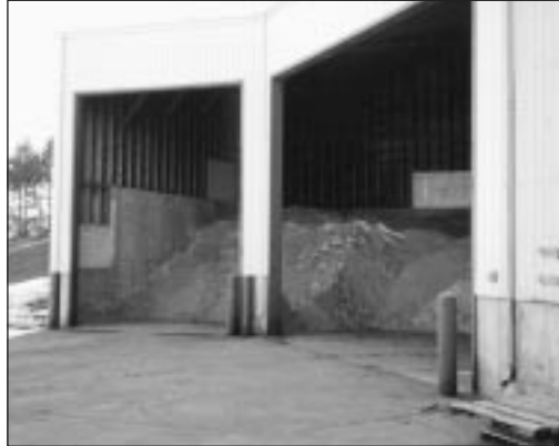
Municipal works yard material storage
