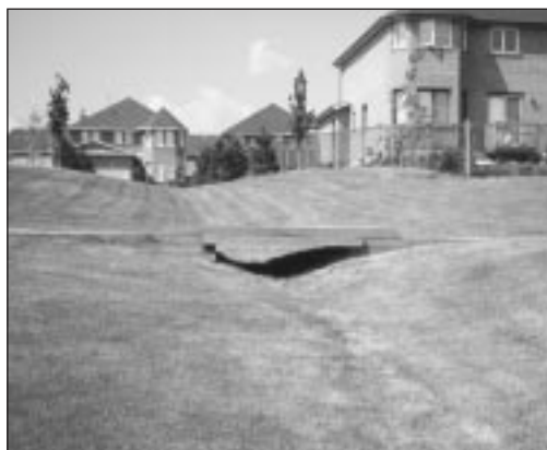
Grassed swales reduce peak flow and trap sediments and nutrients
