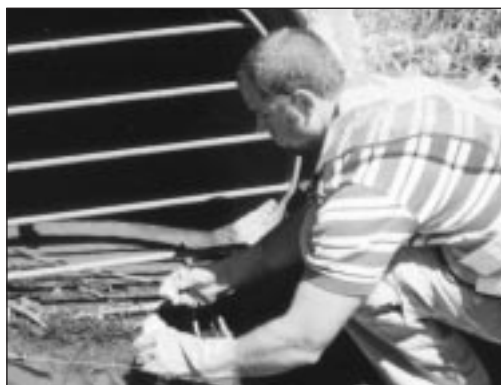
Regular inspection and testing of storm sewers can prevent unwarranted pollution
