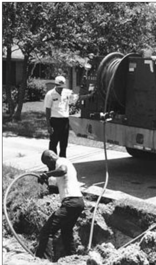
Sewer cleaning crew with a hydraulic jetter trailer
