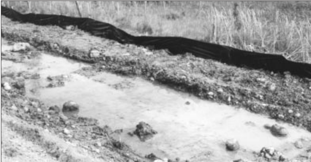
Erosion silt fencing at a construction site
