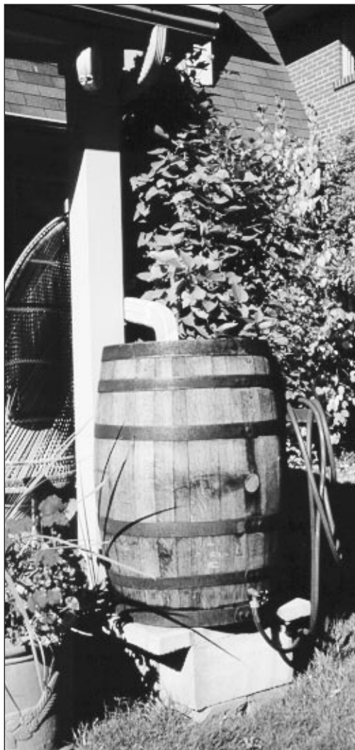
Downspout disconnected and redirected to a rainbarrel
