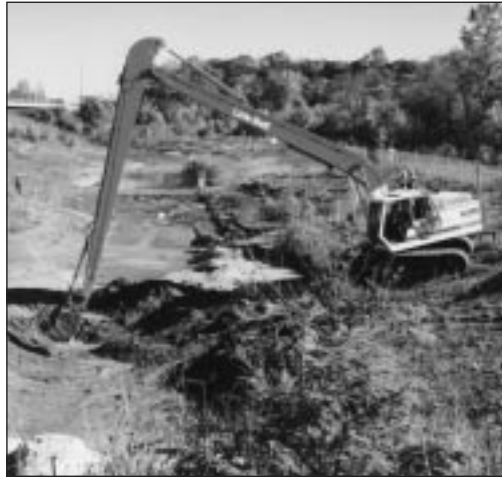
Maintenance and silt removal to promote effective pollutant removal efficiencies
